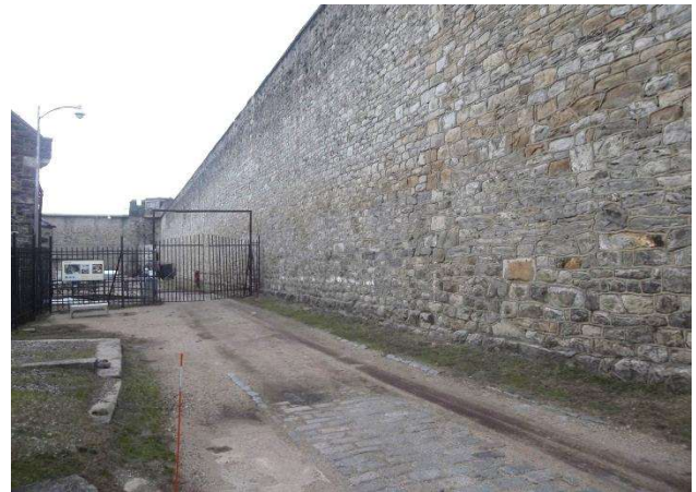
One of the 30 foot high walls (plus 10 foot underground) surrounding the penitentiary.
